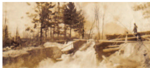
Old High Falls logging dam
